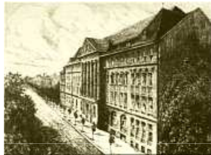
Old ROW Building
